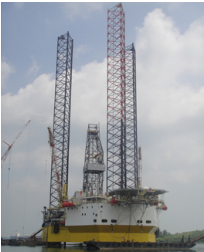
CJ46-X100D Jack-Up Rig, PERRO NEGRO 6. Photo courtesy Drydocks World.
