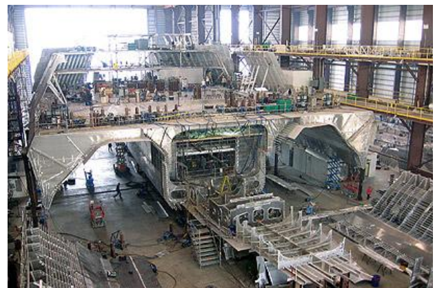
Figure 2 - The LCS under construction at Austral
